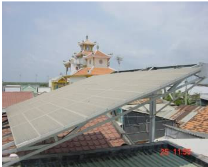
Station fixe solaire hybride Than Ahn Vietnam (500W)
